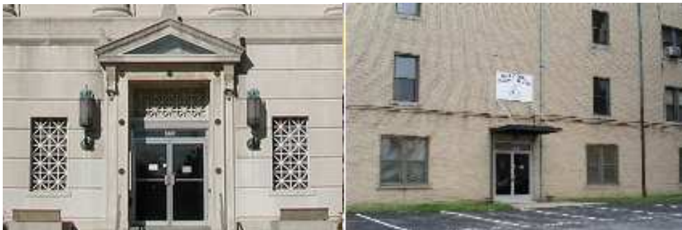
Greensboro Masonic Temple, Market Street Entrance, Parking Lot Entrance
